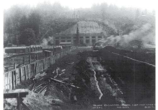
Construction on facilities on the White River
