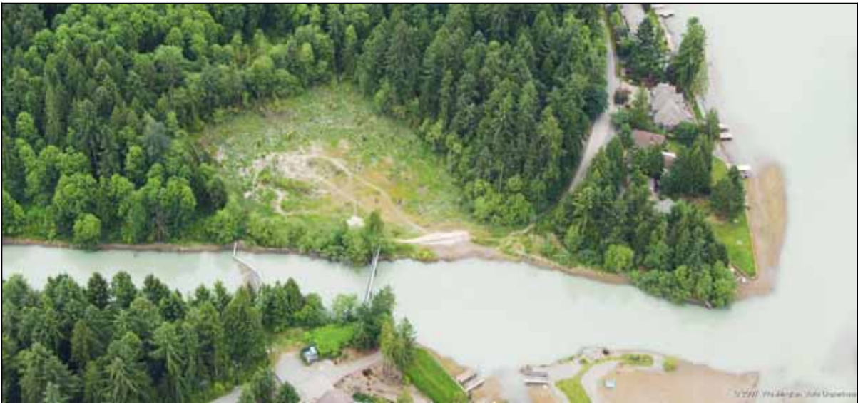
Exhibit 11. View of the south side of the Printz Basin Flume, including associated wetland, as it flows into Lake Tapps.
